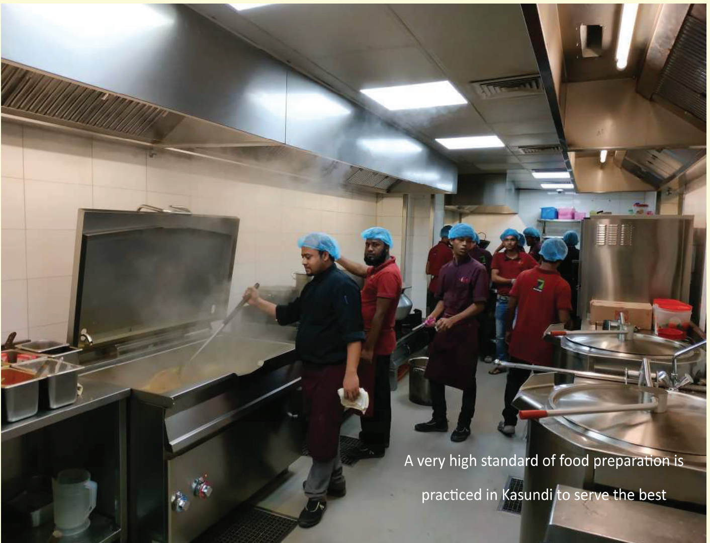
Kitchen 1 of Kasundi Restora Limited Farmgate.
